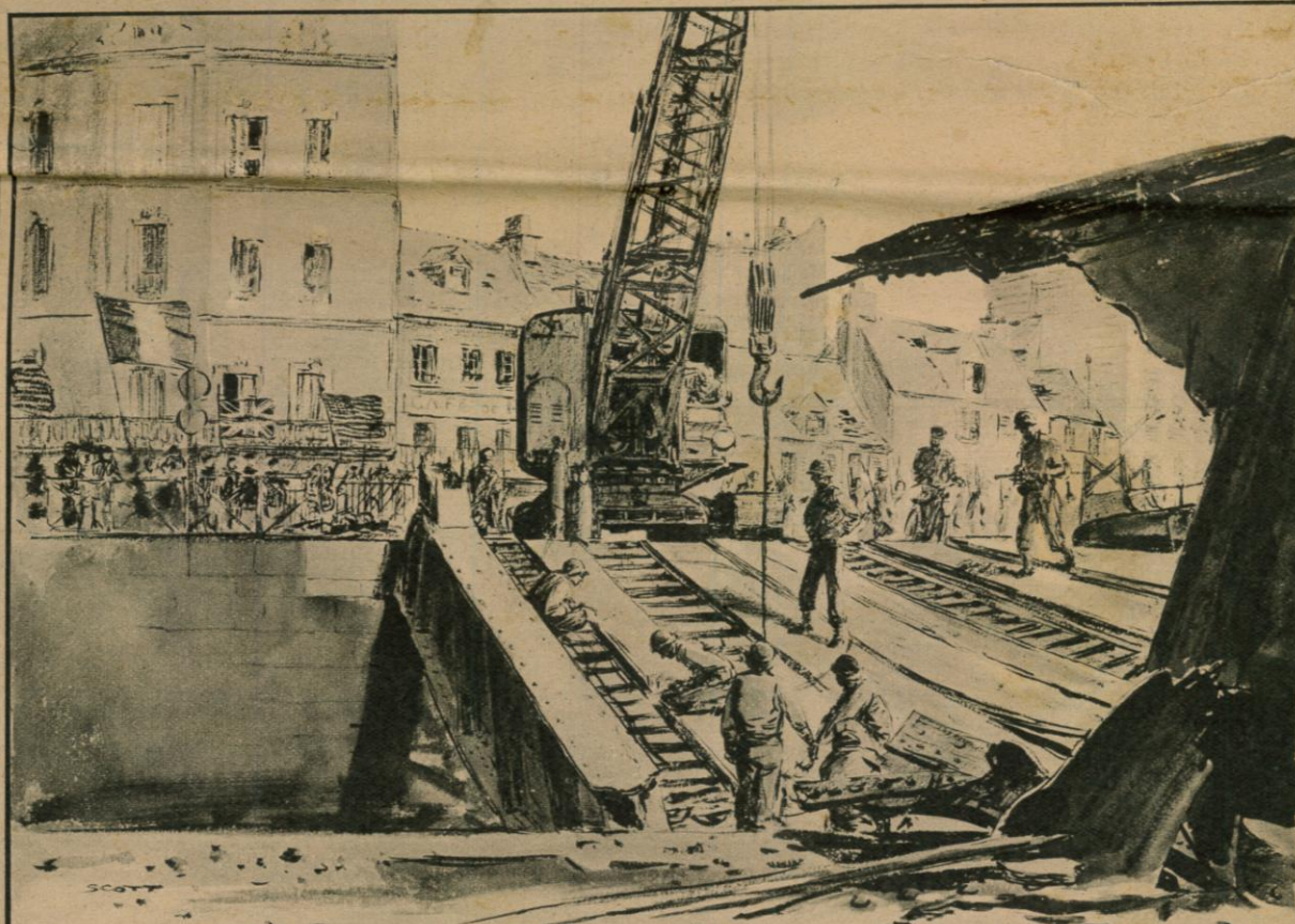
CHERBOURG. Our engineers clearing away the wreckage of a bridge on one of the main streets of the city which had been blown up by the Germans. American, British and French flags were flying from the balcony of one of the buildings across the way. The engineers worked so fast that before noon on the morning I worked on this drawing most of the bridge still visible had been
